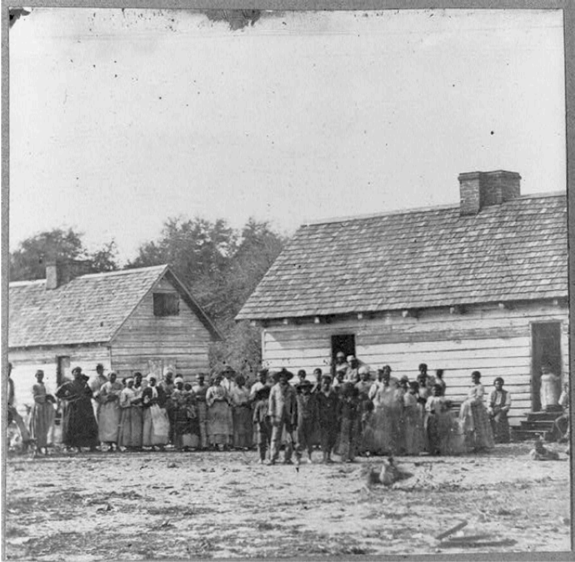
Figure 2.6. Image identified as “Large group of slaves(?) standing in front of buildings on Smith’s Plantation, Beaufort, South Carolina” (b&w film copy negative cph 3b15290, http://hdl.loc.gov/loc.pnp/cph.3b15290 ).
